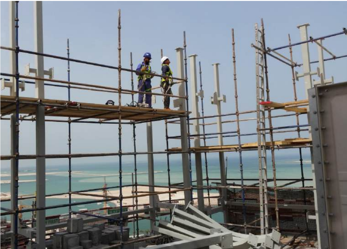
Installation of Steel Structural at AT-MIX-040 Lusail Marina Project : Al Khaliji Headquarters (3B+G+26F)
