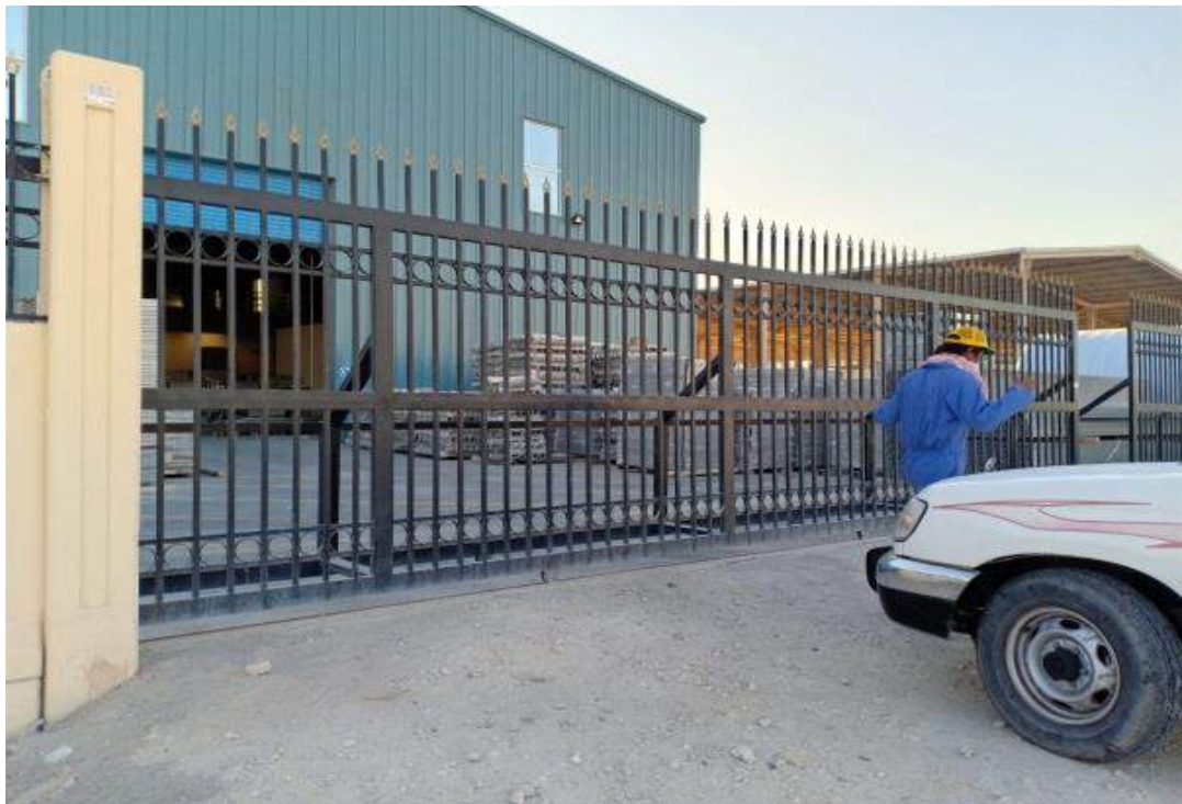
Fabrication & Installation for Steel Sliding System Gate & Boundray Wall At Birkit Al Awamer
