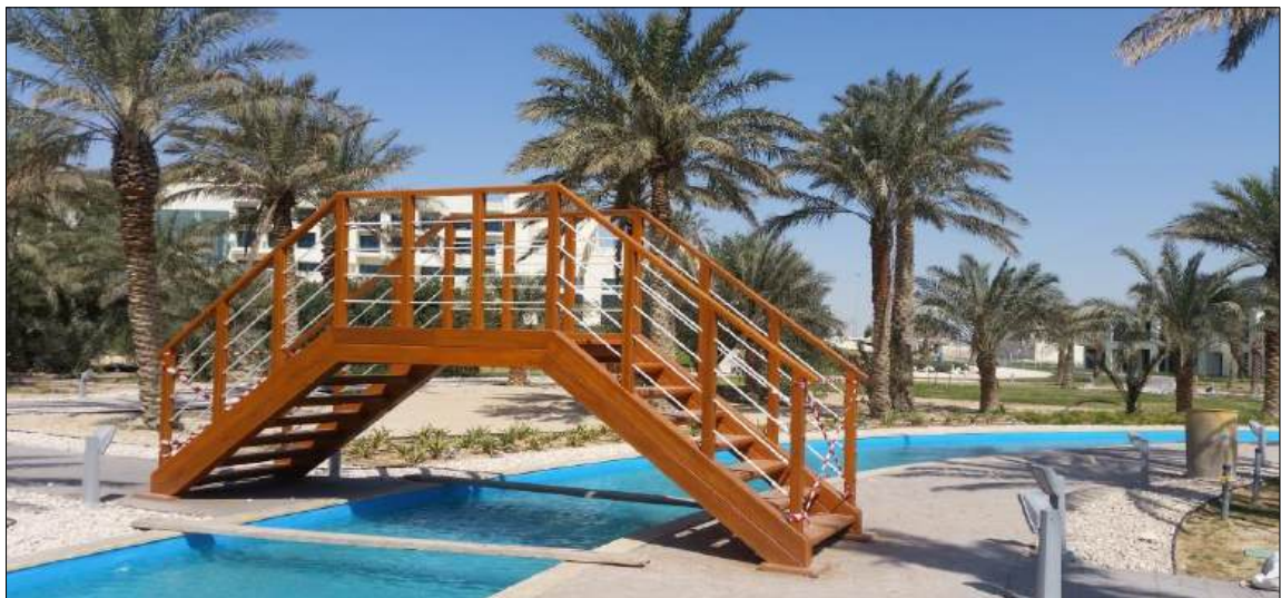
After Installation of Steel Bridges covering by wood at Salwa Resort, Aqua Park
