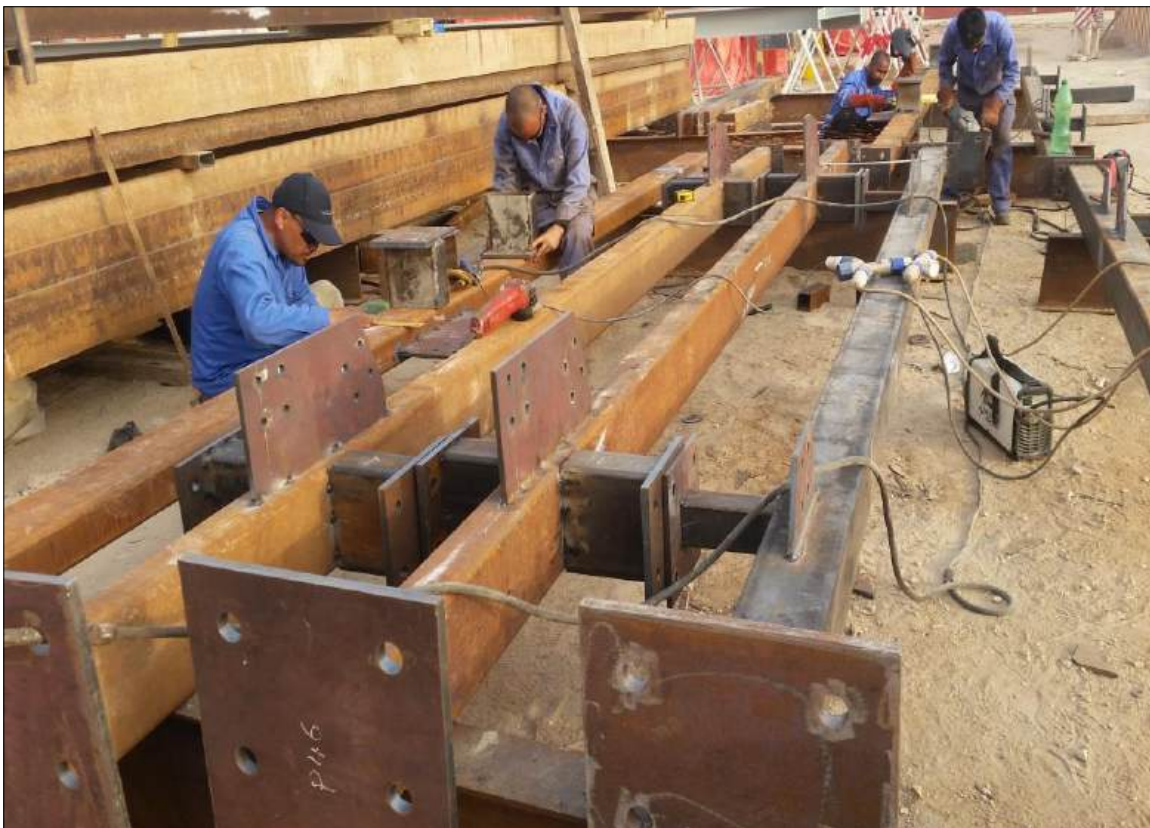
Heavy Steel Structural Fabrication in Workshop for Al Khaliji Headquarters At Mix – 40, Lusail Marina Project
