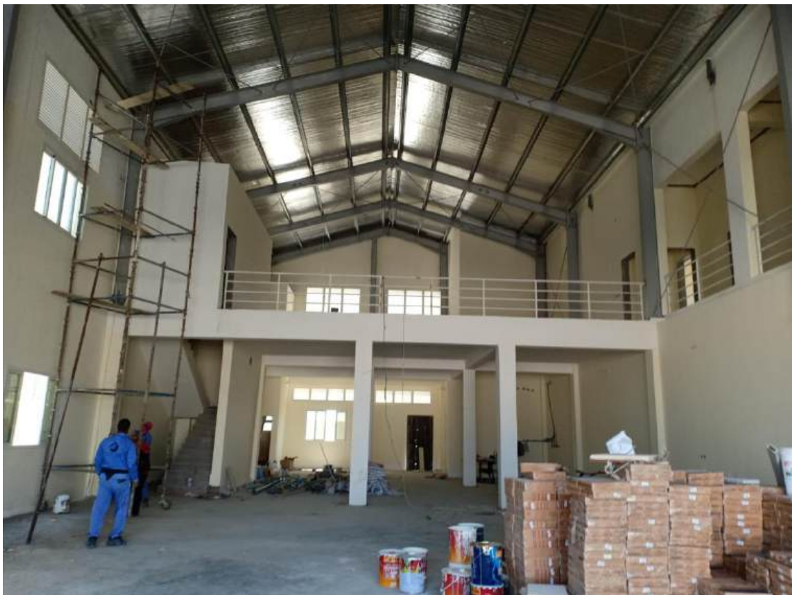
Fabrication & Installation of sandwich panel for roof & Fabrication & Installation of mezzanine floor at Industrial Area Street No. 29
