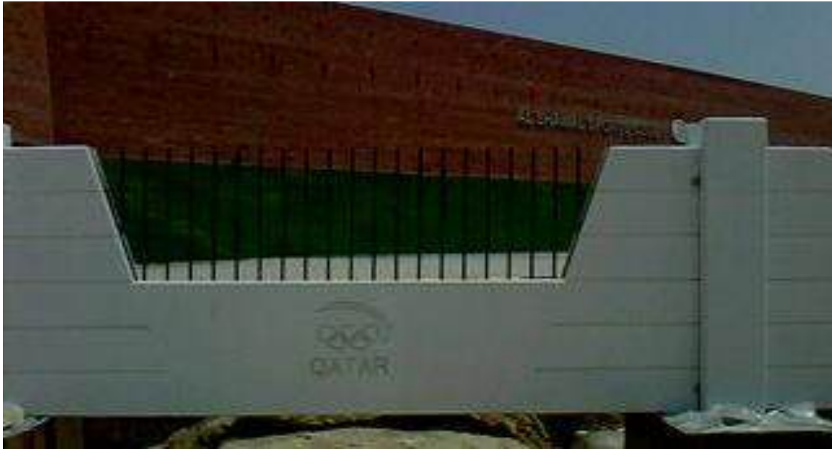
STEEL FENCE AT AL-SHAMAL SPORTS CLUB
