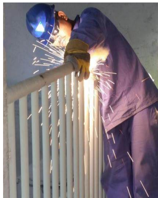
Fabrication & Installation of Steel Pipe Handrail Project : LE Mirage Premium Residential Development (5 Building, 2B+G+7+TECH+P) At Bin Mahamoud, Doha
