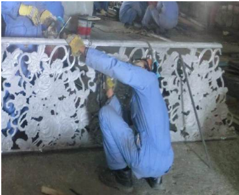
CAST ALUMINIUM HANDRAIL FABRICATION
