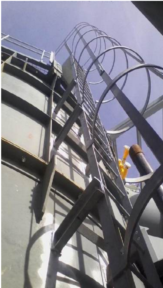
Spiral Steel Staircase & Cat Ladder for Al Farjan Market Stage 2
