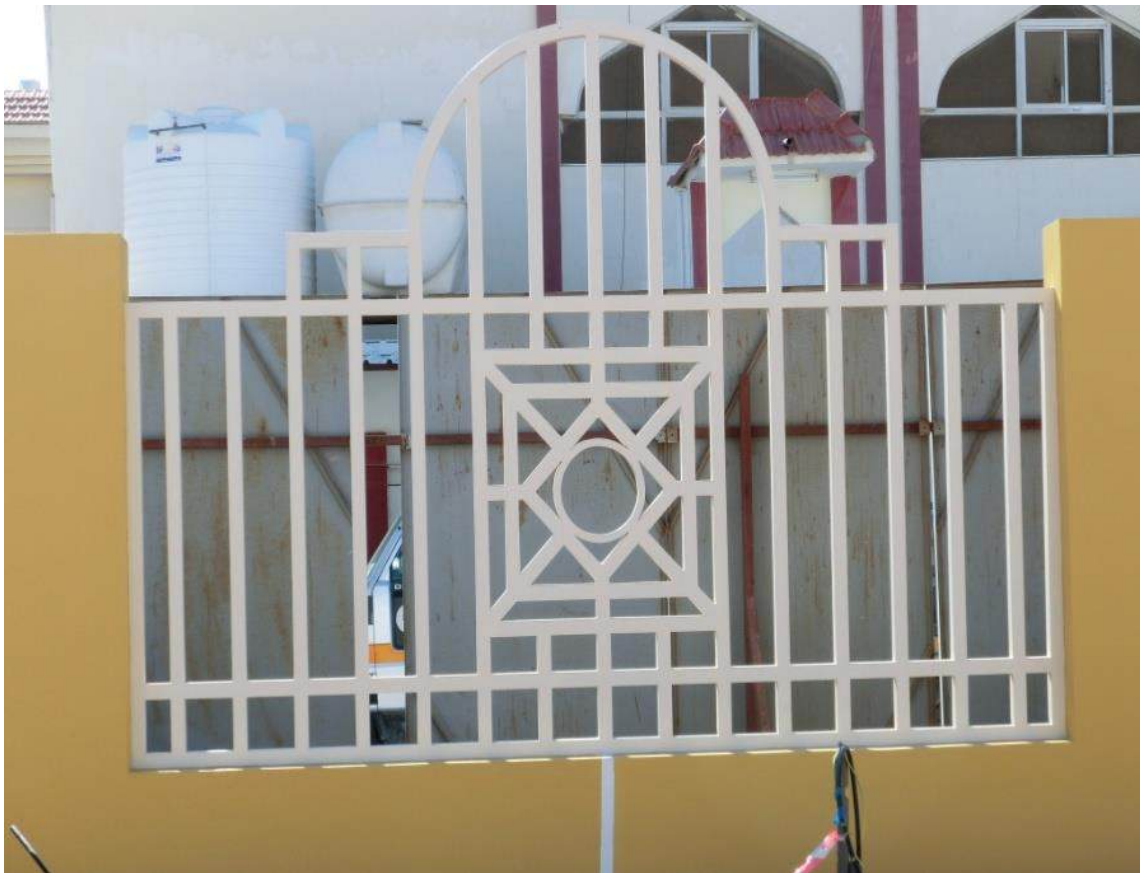
STEEL FENCE AT NUAIIA FOR DOHA MUNICIPALITY
