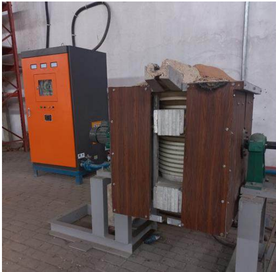
ELECTRIC INDUCTION FURNACE
