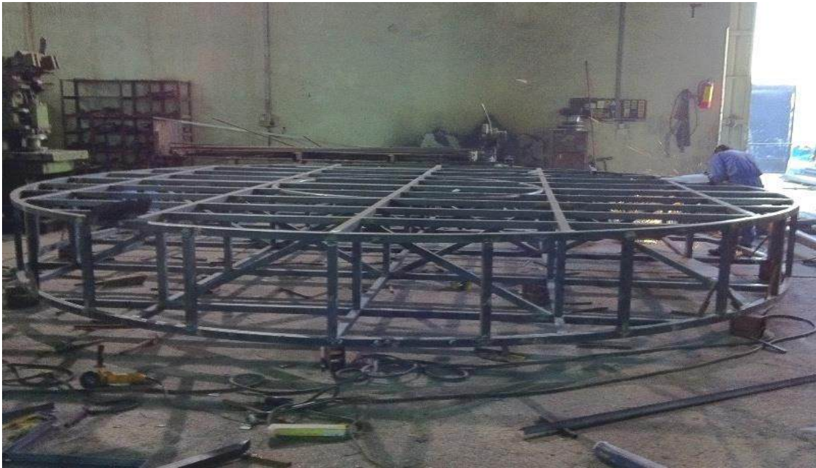
STEEL STAGE FABRICATION (FOR ARAB GAMES 2011)
