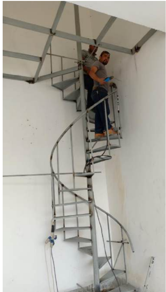
Spiral Steel Staircase & Cat Ladder for Al Farjan Market Stage 2
